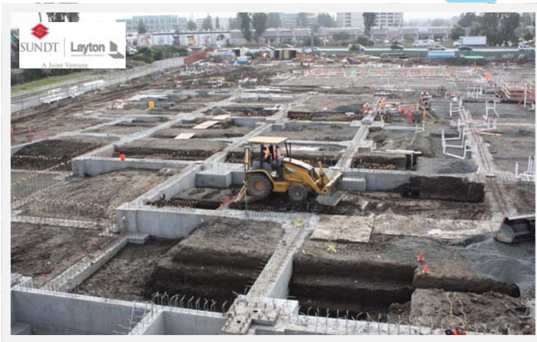
Construction site as of February 12, 2014.
