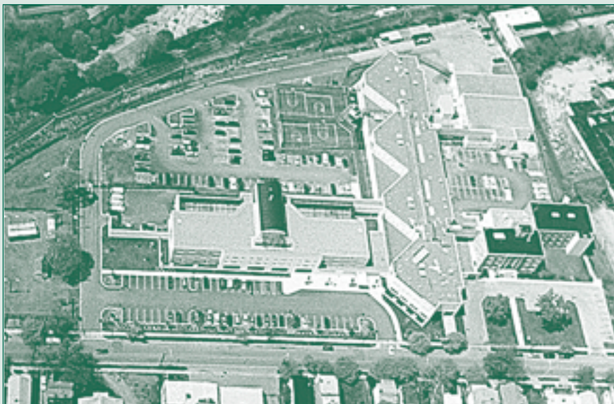
Aerial view of Dutchess County Jail Facility, Poughkeepsie, New York.
